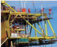
Brownfield Modification & Topside Major Maintenance
